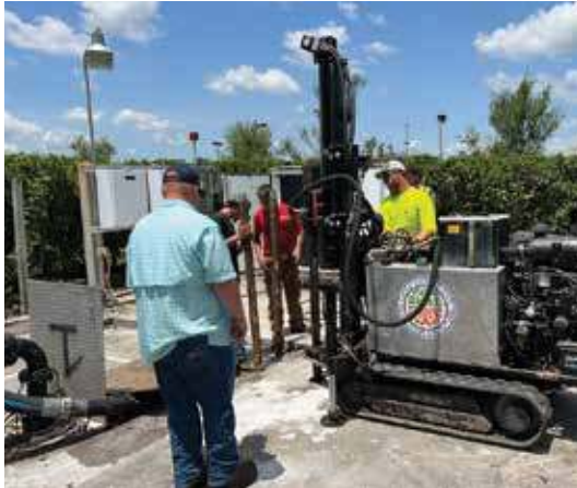
The first injection point on the project was 38 feet below grade and used 710 gallons of chemical grout.
