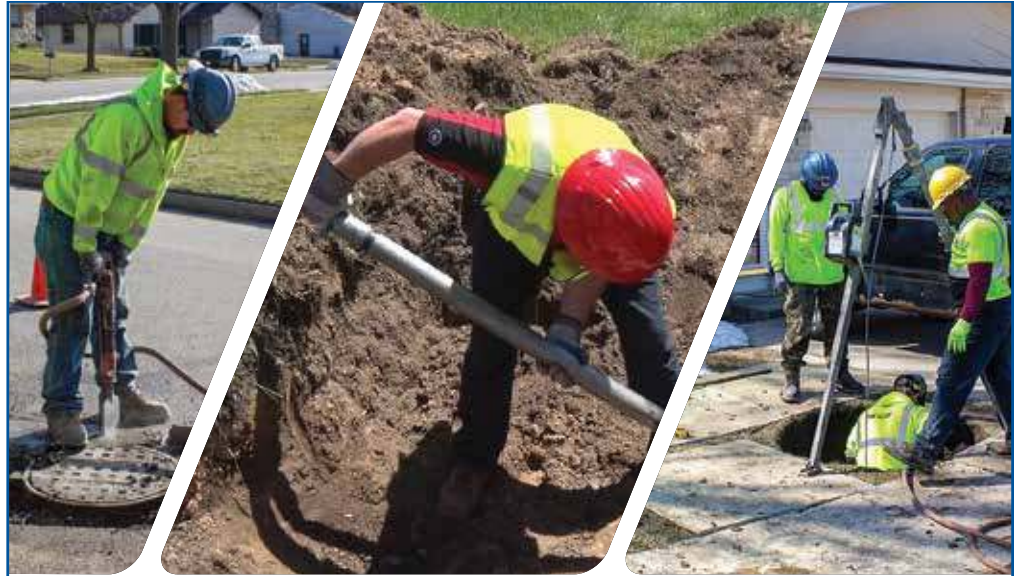
The first injection point on the project was 38 feet below grade and used 710 gallons of chemical grout.
