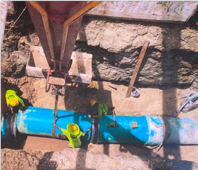
Lift Station 87 subject pipe during original installation
