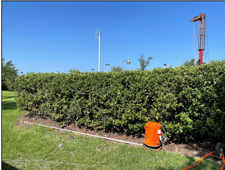
Plate 2 – CSW05 testing on South Side of Lift Station
